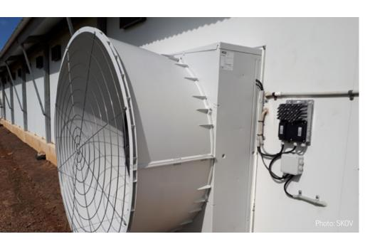
SKOV replaced the existing fans in one of the houses with the new BF 50 BlueFan. Due to the higher ventilation capacity, the number of fans could be reduced from 16 to 13. Comparative tests were then run over five broiler batches.
